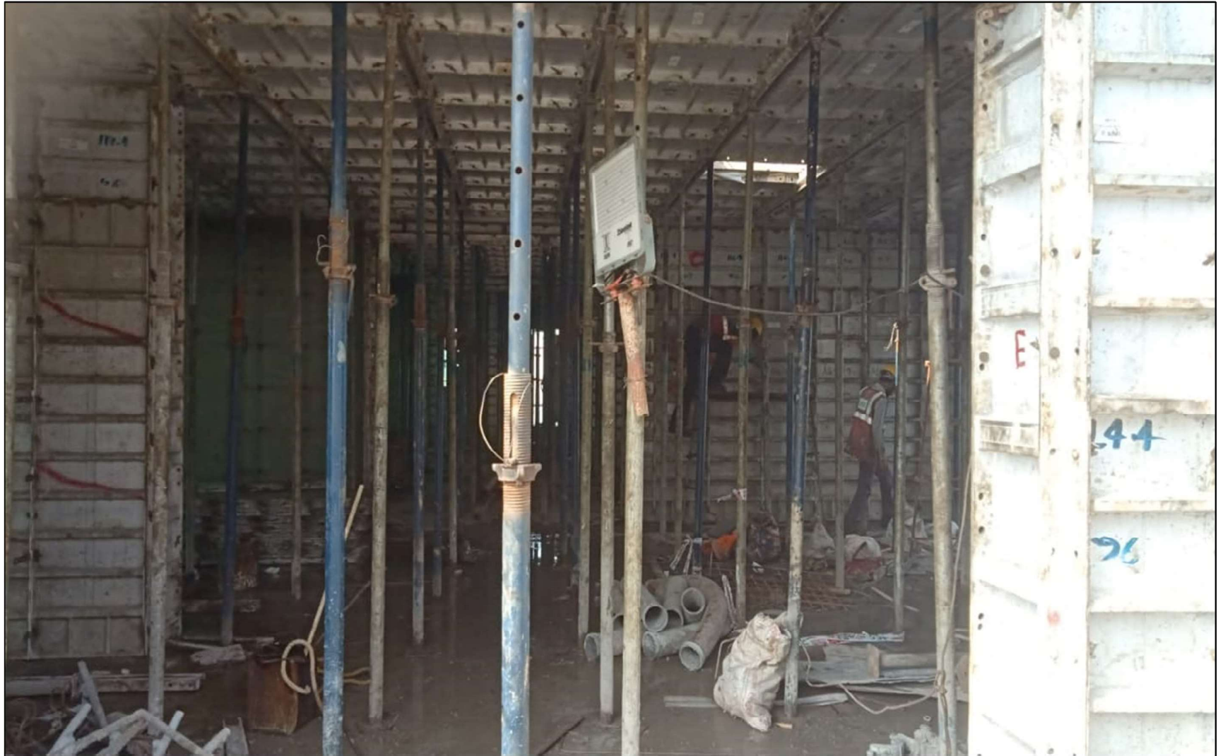
22 nd Floor works under progress
